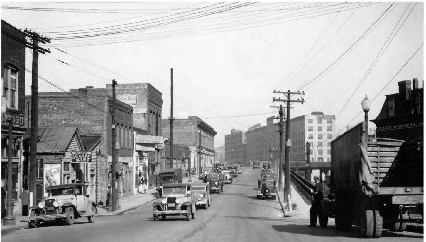
Peters Street Viaduct looking toward the Southern Railway buildings, Atlanta, Georgia c. 1920. Credit: Georgia Department of Transportation.
